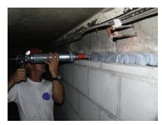
Fire rated sealant being installed to create a rated partition.
